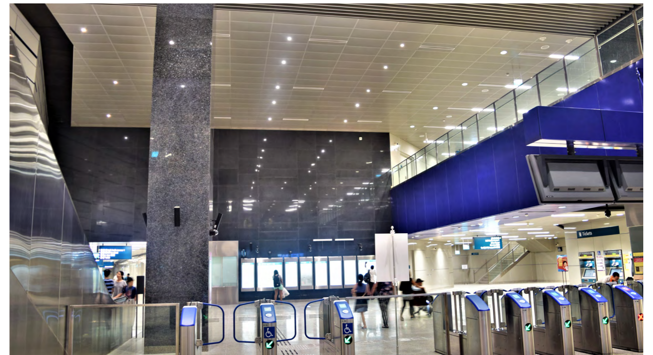
Kaki Bukit MRT station 2,400m 2 of S4 hook-on ceiling, 600 m 2 of 300S-shape strip ceiling, 600 m 2 of POLYLAM® TYPE X vertical baffle system.
