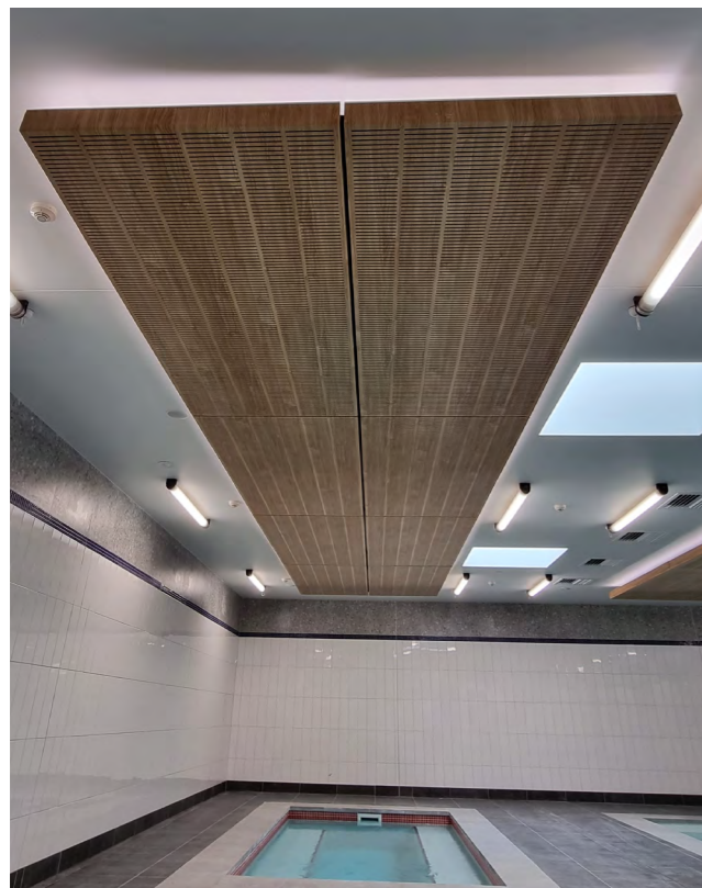
Newcastle Knights Centre of Excellence durlum's S7 bespoke wood grain ceiling with slotted perforations.
