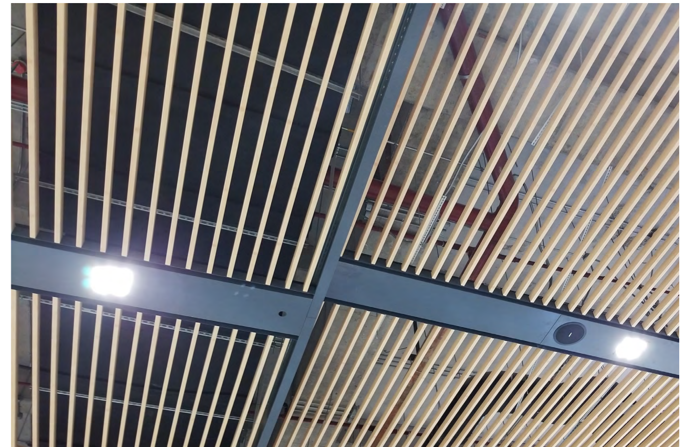
Mactan-Cebu Airport, Philippines 20,000m 2 of POLYLAM® TYPE X vertical baffle system, S4 RHOMBOS expanded metal ceiling, Binnacle & Retail Cladding, Trellis.
