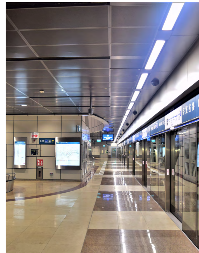
Geylang Bahru MRT station 200m 2 of S4 RHOMBOS and 3,900 m 2 of S4 hook-on ceiling.
