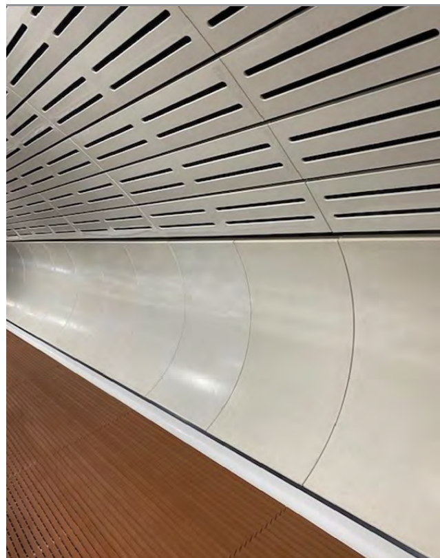
Victoria Cross Station, Sydney Metro 7,000m 2 of durlum's bespoke designed S7 metal ceiling installed on curved cavern ceiling and walls.
