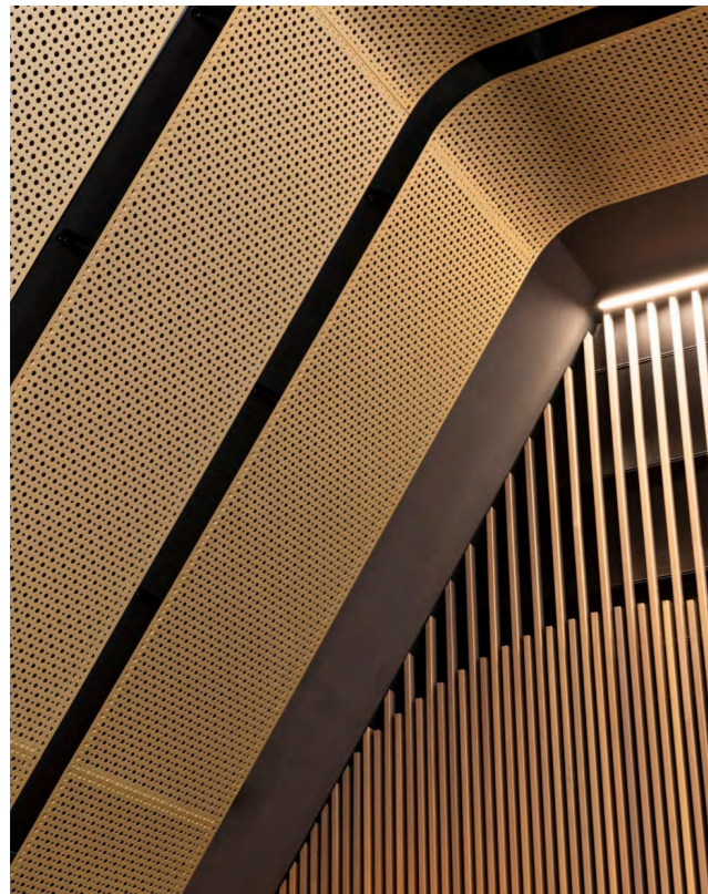
MARVEL Stadium durlum custom u-shaped anodised canoe rafts 300LM and durlum custom s-shaped metal raft ceilings.
