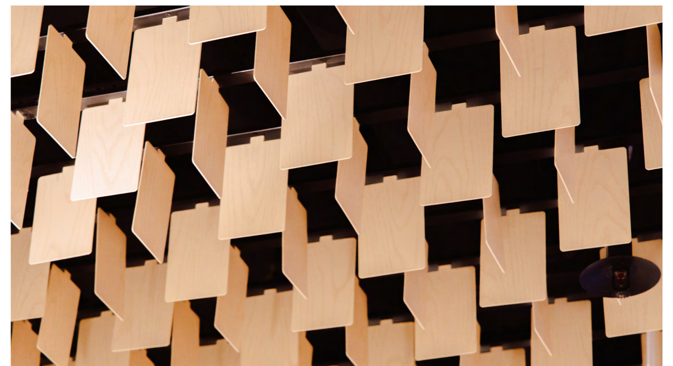
Castle Towers Shopping Centre 4,800m 2 of durlum's LIVA open cell louvre ceiling system with bespoke timber and bright pastel finishes.
