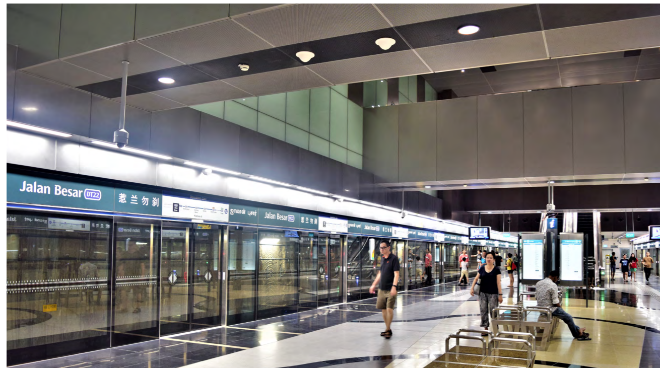
Jalan Besar MRT Station 4,400m 2 of S4 hook-on ceiling, 630 m 2 of 300S strip ceiling.
